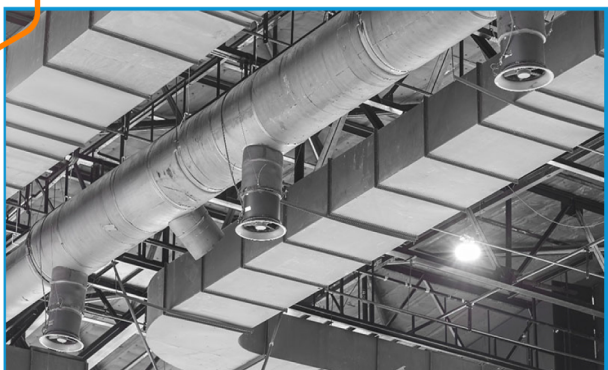
OPEN DUCTING SYSTEM
